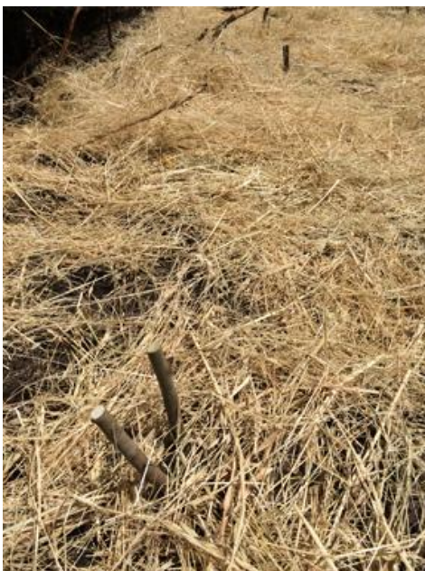
Native seed and willow stakes were planted during construction.
